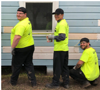
Volunteers from Cummins show off their siding repair skills.
